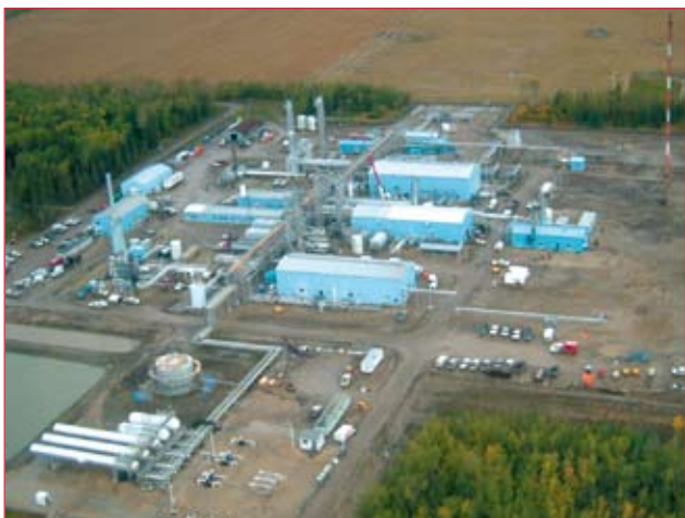
Figure 1. Wembley gas plant.
